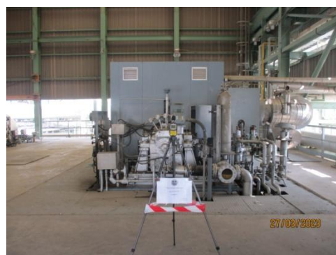
Propylene Compressor (R-650)
